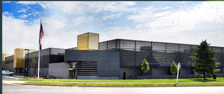
RagingWire VA1 Data Center, next door to Old Ox Brewery
